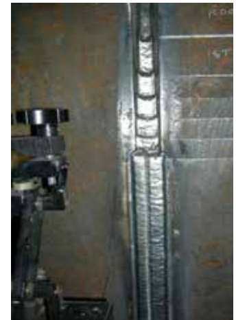
Mechanized welding of LNG storage tanks with BÖHLER NIBAS 625 PW-FD (ENiCrMo3T1-4).
