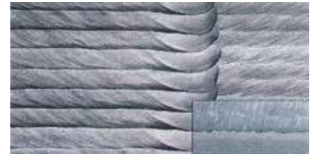
Cladding with Böhler CN 23/12 Mo-FD (E309LMoT0-4/1) for the 1 st and BÖHLER EAS 4 M-FD (E316LT0-4/1) for the 2 nd layer. Results in very uniform ferrite levels.
